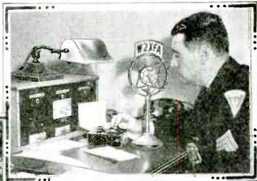
Sgt. Conroy using the portable microphone. All equipment, except the control panel, is located under the rear deck. Besides the main operating room at Headquarters, two receivers at remote points are used to provide reliable communication.
